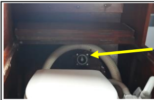
W-class – behind the toilet in the forward cabin
